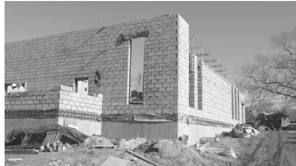
...CMU work at rear of apparatus bay
