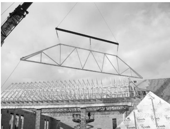
...Swinging large apparatus bay trusses
