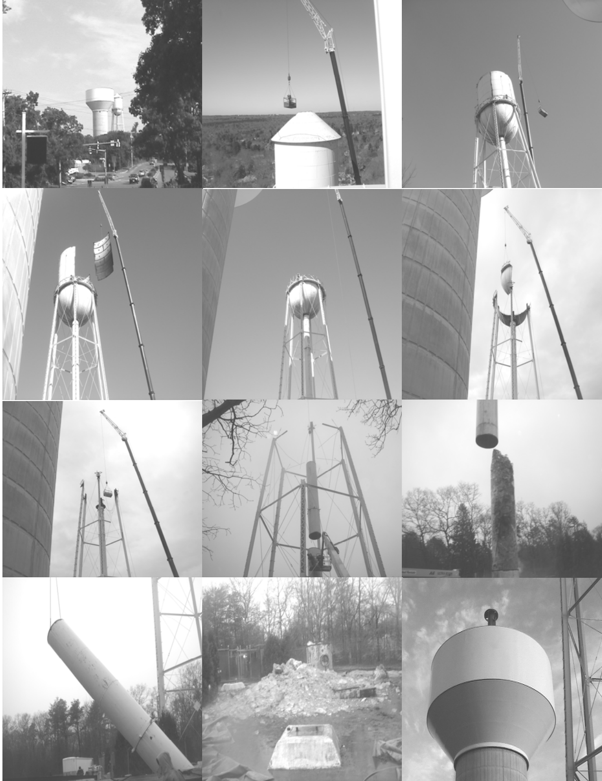
REMOVAL OF OLD WATER TANK
